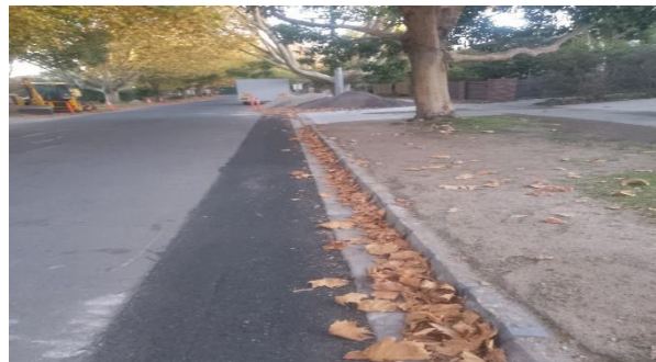
Bowen Street Camberwell 2024 bluestone kerb and channel reconstruction
