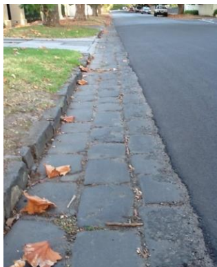
Three pitcher kerb and channel Victorian era 1880s-1900s Sackville Street Kew
