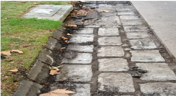
Bowen Street Camberwell 2024 bluestone kerb and channel reconstruction
