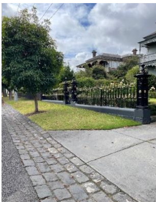
Bluestone spoon drain channel Victorian era 1850s-1870s Neave Street Hawthorn
