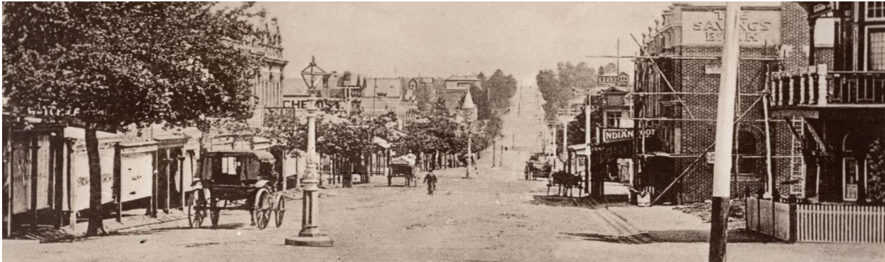
Bluestone Kerb and Channels in Burke Road Camberwell 1910
