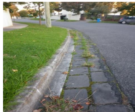
Concrete kerb and bluestone Interwar era 1919-1939 Hyton Crescent Kew
